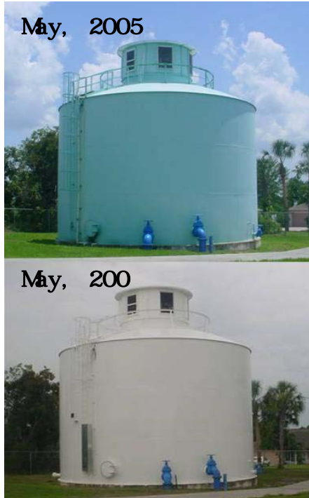
Storage Tank repairs and repainting completed May 19, 2006
